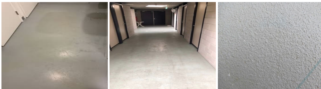
Foto 1: Coating intact, lichte vervuiling
